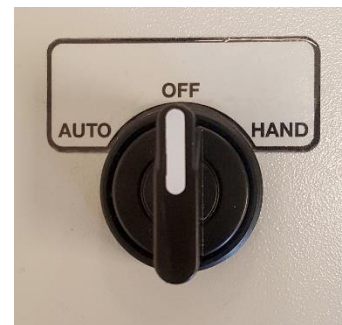
Figure 4-1: Example of a HAND/OFF/AUTO (HOA) Switch
